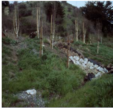
Grassed drainage area.
