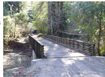
**Steel Bridge installed on Soquel Creek to replace a ford crossing.**
