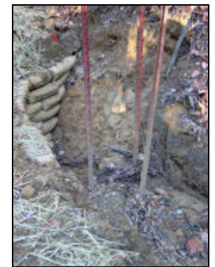
Debris alignment racks ("trash racks") on culvert inlets help catch woody materials and vegetation that can plug culverts.
