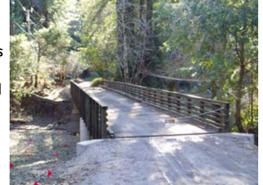
Steel Bridge installed on Soquel Creek to replace a ford crossing.
